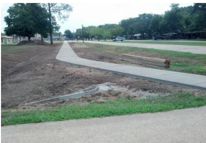
Bowie Elementary School
