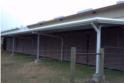
Ag Barn renovations
