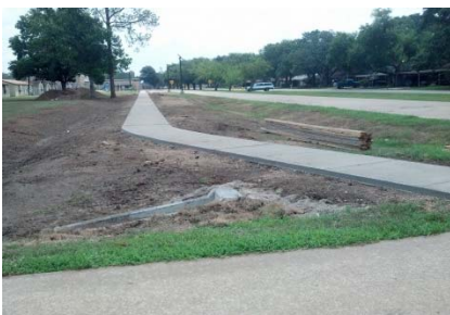
Bowie Elementary School
